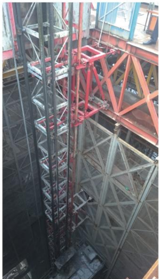
单导轨上爬模顶部 Single mast going to the top of the climbing formwork.
