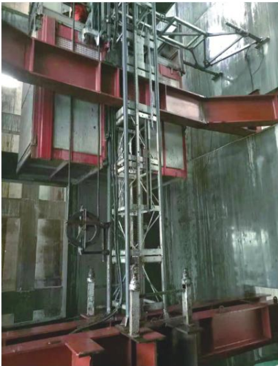
井道内升降机基础转换 Foundation conversion for outdoor lifts. 东莞国贸 428m
