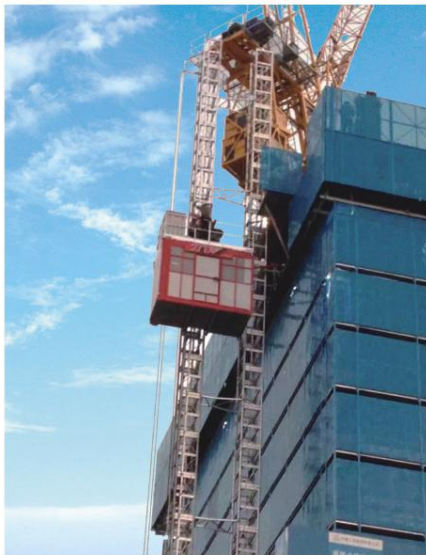
双导轨上爬模顶部 Double masts going to the top of the climbing formwork. 珠海横琴国际金融中心 338m
