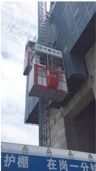
单导轨上爬模顶部 Single mast going to the top of the climbing formwork.
