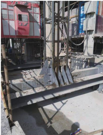
室外升降机基础转换 Foundation conversion for outdoor lifts. 重庆来福士 350m
